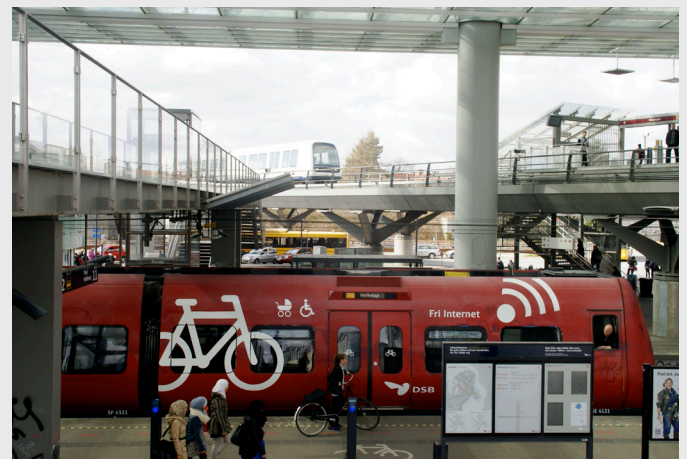
Local railway and metro integration, forming a more convenient transportation hub. (Photo: Daniel Sparing, Creative Commons)
